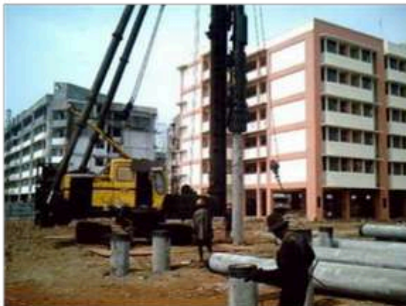
Gambar 2 Alat pancang Jack-in Pile
